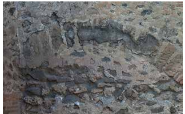
Fig. 15. Upper part of the relieving arch housed in the boundary shared with the atrium of Domus V 1,3 (Room 2). To the left is the interior separation between the rear rooms of Fullonica V 1,2 (Rooms 4 and 5), functioning as support for the west springer of the relieving arch. Photograph: Hans Thorwid.
