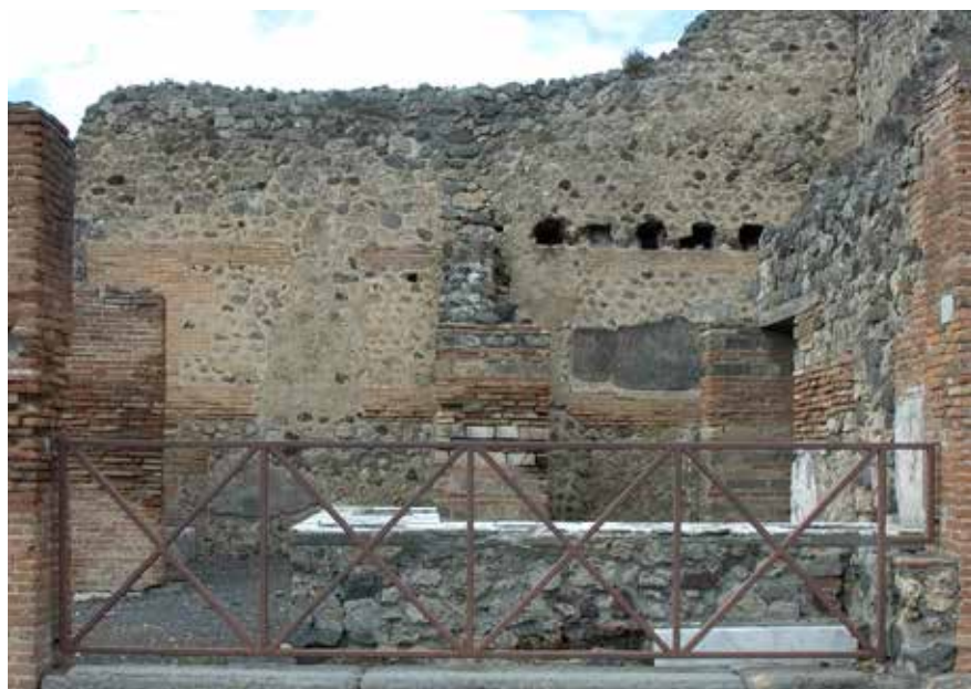
Fig. 17. Interior view of Thermopolium V 1,1.32 showing the Long Boundary, here functioning as north delimitation of Rooms 6 and 7. Note the characteristic incertum-masonry interspersed with courses of bonding tiles and the brick-faced concrete of the east end of the Long Boundary. In front further brick-masonry techniques used for inner separations and for the corner pylon of the façade (left in picture). Photograph: Hans Thorwid.
