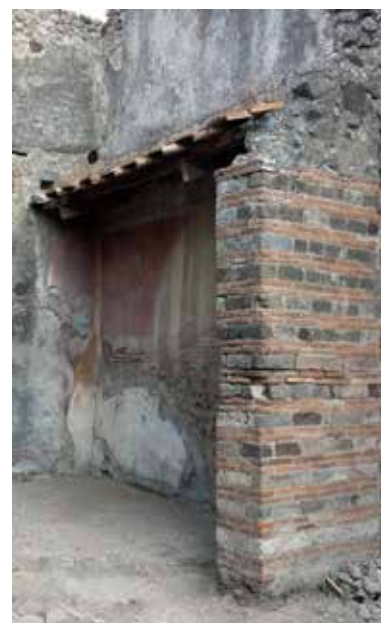
Fig. 18. Brick-and-block-built separation between front and rear rooms of Taberna V 1,31, Rooms 1 and 2. The modern shelter roof protects decorations which may indicate some public function, perhaps a retail shop. Photograph: Hans Thorwid.
