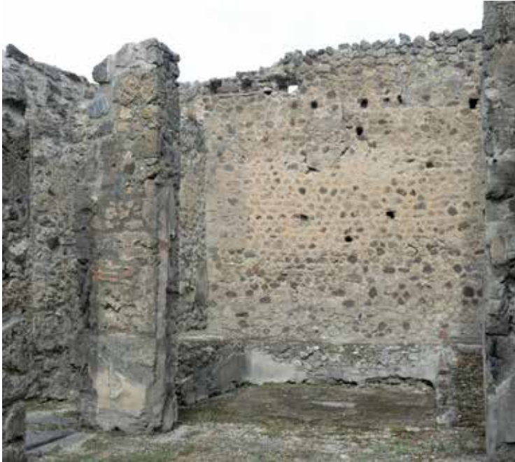
Fig. 27. The rainfall-collecting area situated north-east of the atrium in Domus V 1,3, Room d, view from Room 4, triclinium of Domus V 1,3. Note the three beam holes to the left in the rear wall demonstrating the former presence of a roof, and east of this, a lower row of lesser beam holes suiting a shelter roof. Photograph: Hans Thorwid.
