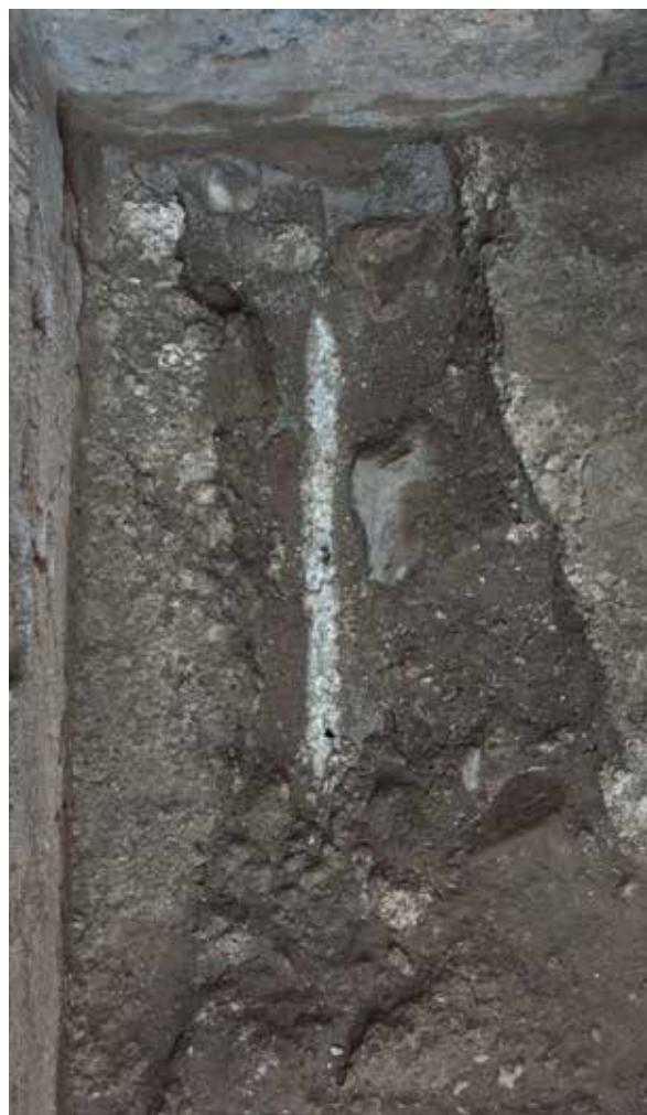
Fig. 34 (left). Domus V 1,3, Room b: service corridor. The floor has been broken to house the pipe for pressured water entering Domus V 1,3 from the House of the Bronze Bull. Photograph: Hans Thorwid.
