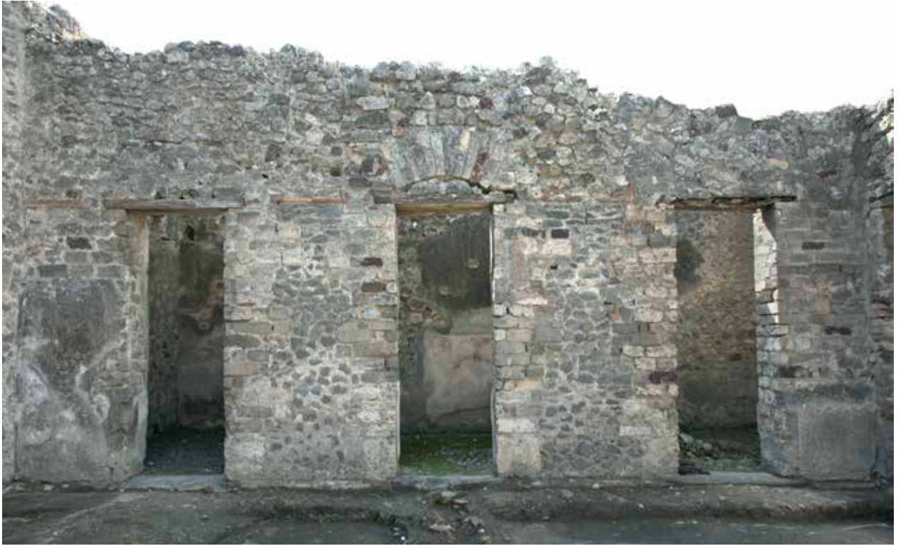
Fig. 42. West wall of the atrium of Domus V 1,3, Room 2. The tuffelli-framed doorways mark a remake and strengthening of the wall. Photograph: Hans Thorwid.
