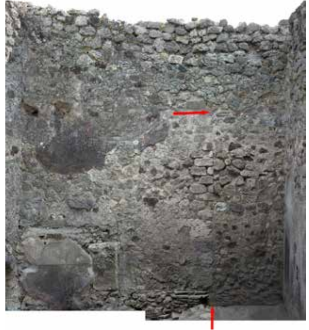
Fig. 33. House of the Bronze Bull: walled-off doorway, closing the passage to Domus V 1,3. Arrows highlight the tufelli frame of the former opening. V 1,7.9 Room i, south wall. Feature highlight: Henrik Boman. Photograph: Hans Thorwid.
