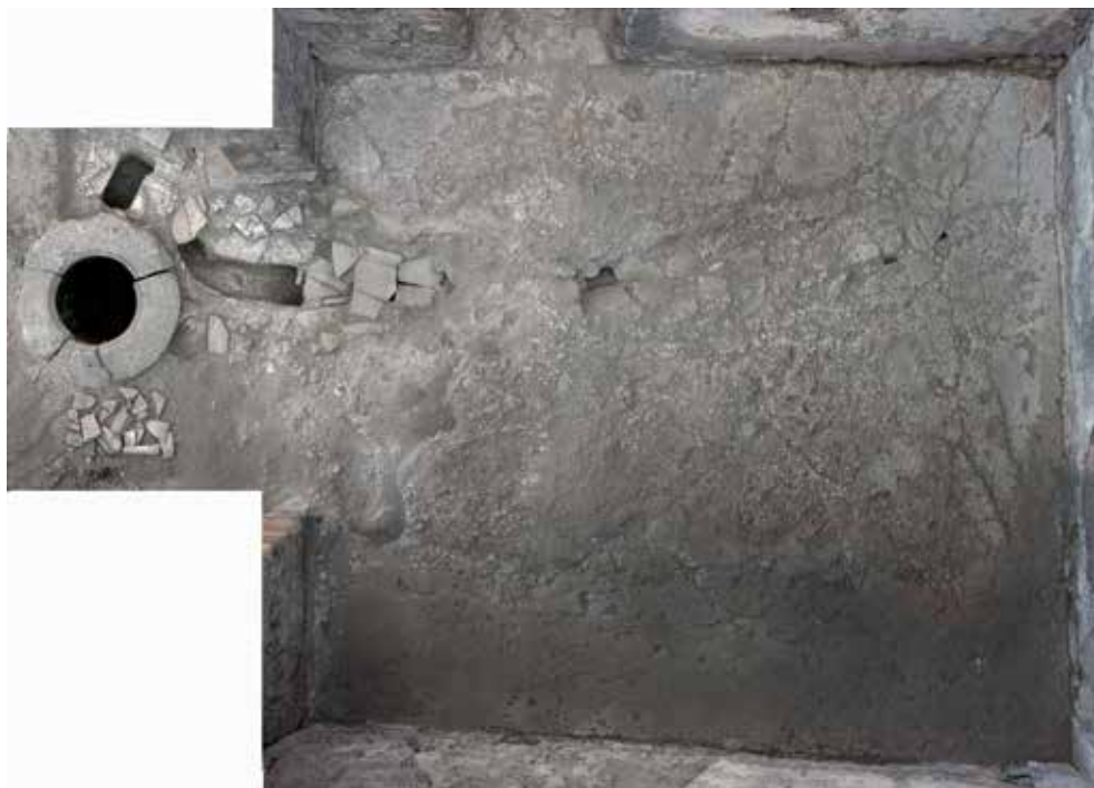
Fig. 19. Plan view of the cocciopesto floor of the main rear room of Taberna V 1,31, Room 2. The floor abuts the walls on all sides and is covered by extant wall plaster in the south-east corner. Note the drain channelled beneath; after making a turn for depositing unwanted elements, it enters the shaft of the cistern. Photograph: Hans Thorwid.
