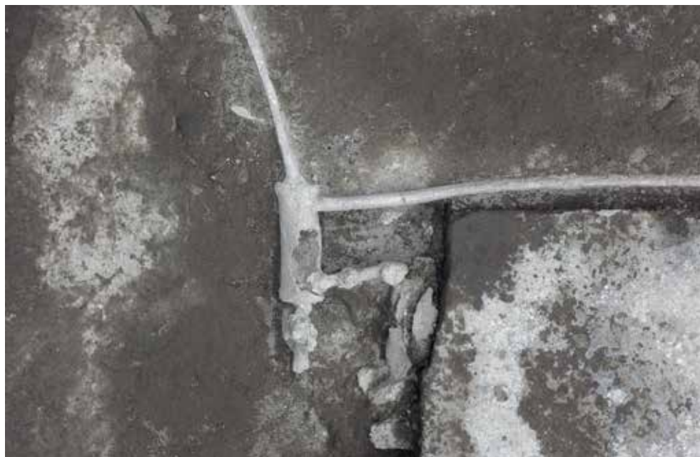
Fig. 26. Domus V 1,3 Room 2 (atrium) . Pipes and distribution box by the north-west quoin of the impluvium. Note the two taps, and the lead cap strengthening the 90° dive of the middle pipe. Photograph: Hans Thorwid.
