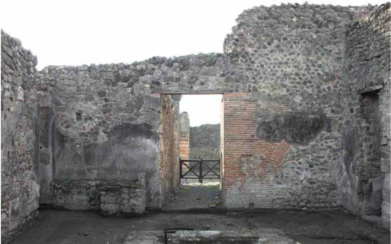
Fig. 12. Domus V 1,3. South wall of the atrium (Room 2) with relieving arch and extensive brick-and-concrete buttressing. Photograph: Hans Thorwid.
