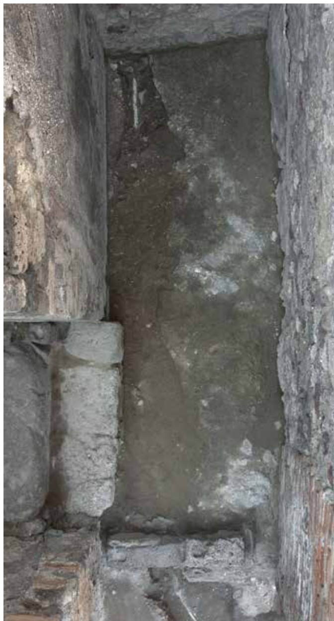
Fig. 34 (left). Domus V 1,3, Room b: service corridor. The floor has been broken to house the pipe for pressured water entering Domus V 1,3 from the House of the Bronze Bull. Photograph: Hans Thorwid.
