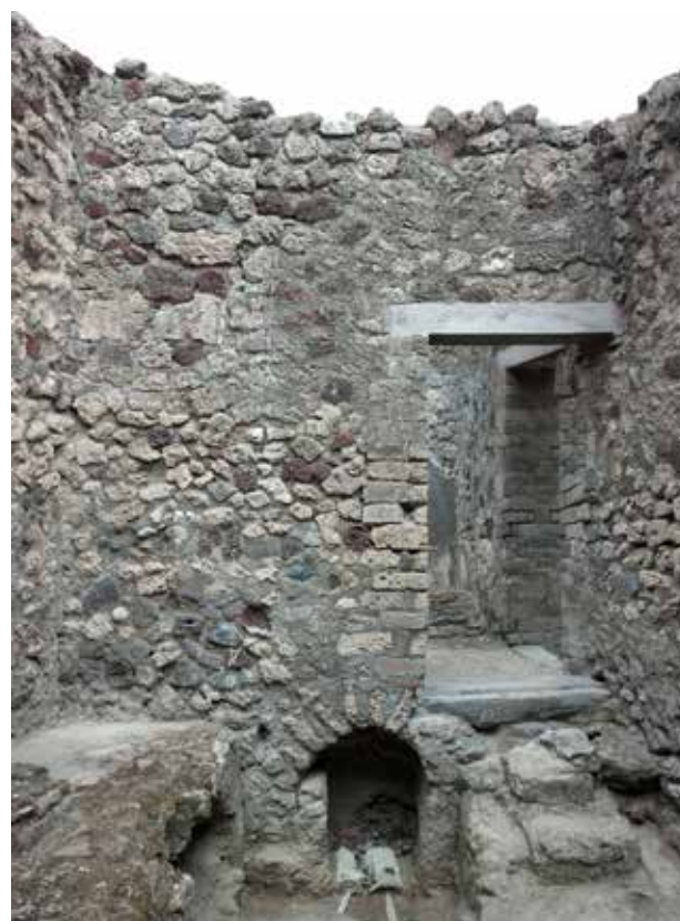
Fig. 24. Kitchen of the House of the Bronze Bull (V 1,7.9, Room l). East side of the room containing a niche for the pair of water-distribution boxes and a staircase leading to the same level as the main part of the West Wing and the peristyle area of the house. Photograph: Hans Thorwid.
