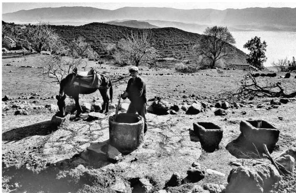
Fig. 3. A cistern. The sedimentation tank is just visible at the front edge of the cistern apron. Photograph: © Tobias Schorr, www.methana.com .
