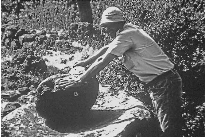
Fig. 4. A crusher, the traditional uses of which included crushing pottery for making hydraulic cement. Photograph: Hamish Forbes.
