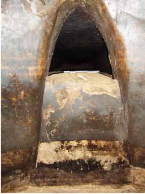
Fig. 9. Kerameikos bath, second phase, Z 16, separation wall. Photograph: Jutta Stroszcek.
