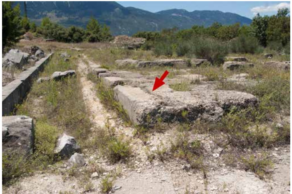
Fig. 6. The trace of weathering of the toichobate on the extant foundation of the cella. View from the east, viewpoint shown on Fig. 9. Photograph by C. Kanellopoulos.
