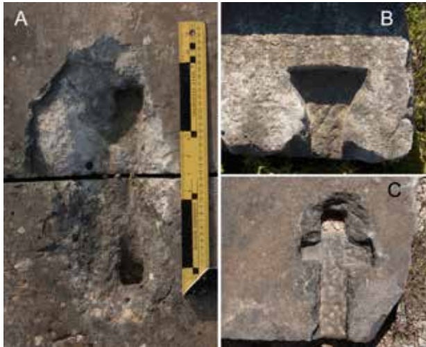
Fig. 14. Clamp sockets a. from the krepis second step; b. from a block in the depot; c. from the ramp of the Temple of Zeus. Photographs by C. Kanellopoulos.
