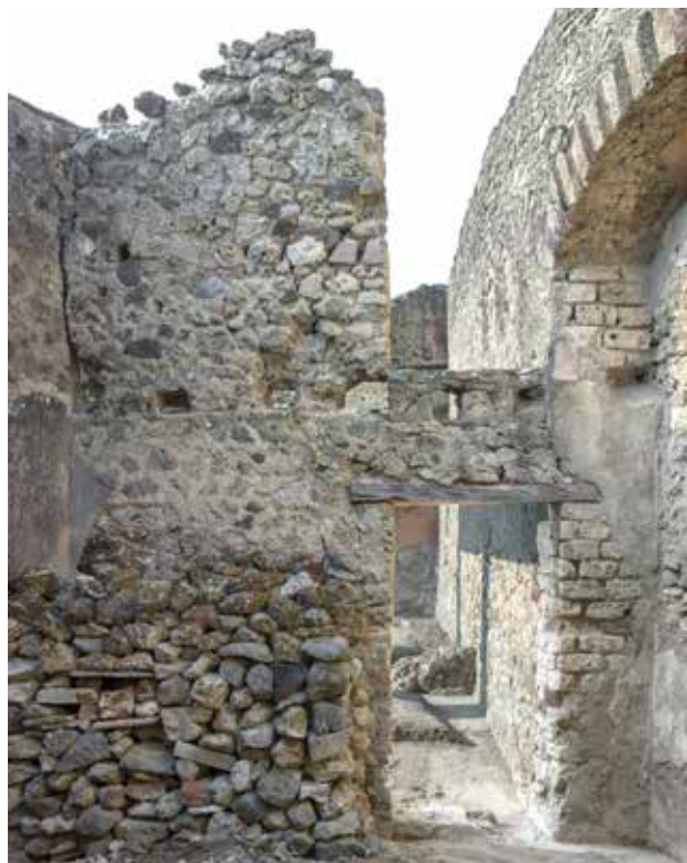
Fig. 23. East insula perimeter with added inner wedge-shaped wall-shell revetment in small tufa blocks. House of the Greek Epigrams, north wall of room V 1,18k. See also the ground-plan produced by means of horizontal sectioning, Fig. 9. Photograph: Hans Thorwid.
