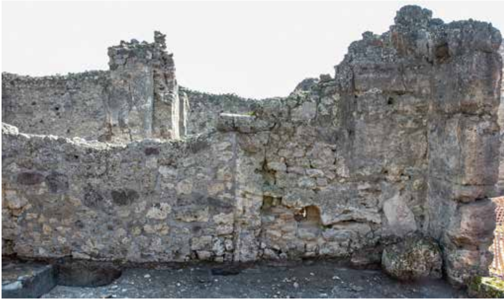
Fig. 21a. Walled-up doorway in boundary separating V 1,13a from V 1.14i, viewed from the north side of the boundary (the caupona side). The limestone pillar is understood as the west door-jamb. The east jamb is covered by modern restoration work (covering most of boundary left of the jamb in the image), but visible on the other side of the wall (Fig. 21b). Photograph: Hans Thorwid.
