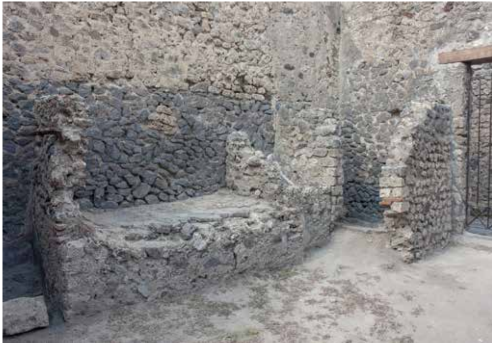
Fig. 7a. View towards the north-east corner of the North House of Caecilius Iucundus (kitchen and latrine, V 1,23n). Homogeneity of texture of the lava incertum characterizes the north boundary and the east perimeter. Photograph: Hans Thorwid.
