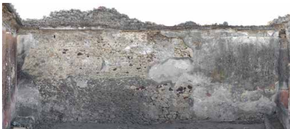
Fig. 3. East part of the boundary between the House of the Greek Epigrams (V 1,18.11.12) and the North House of Caecilius Iucundus (V 1,23.10) displayed as a wall-string. South elevation with inner divisions cropped away. The arrows indicate two abrupt changes in masonry texture. To the right, the wall “wound” indicating a robbed boundary return, to the left a change in masonry. Visualization: 3DHOP software. Feature highlights: Henrik Boman.
