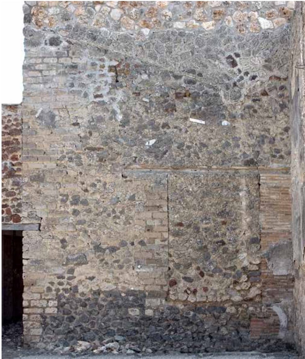
Fig. 27. Opus incertum masonry supported by tufelli framework. West façade towards courtyard V 1,23l of the east triclinium (later V 1,26o). To the right, later brick repair replacing the original southern tufelli frame of the blocked window. Photograph: Hans Thorwid.
