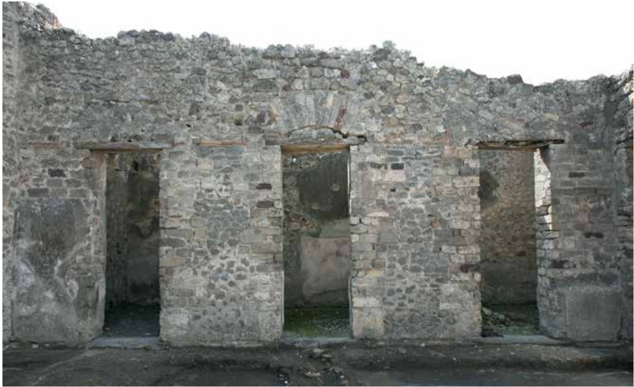
Fig. 29. The imperial-age tuffelli-framed door-ways leading from the atrium towards the cubicula of House V 1,3, west wall of atrium V 1,3,2. Photograph: Hans Thorwid.
