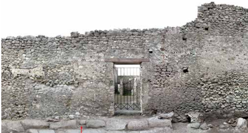
Fig. 7b. Façade towards the east rear street (Vicolo di Cecilio Iocundo). The perimeter wall of the North House of Caecilius Iucundus turns 90° to continue as the north border of the East Property as demonstrated in Fig. 7a. The façade of the House of the Greek Epigrams (to the right) uses stones of lighter colour. The arrow indicates the former extent of a putative shop-opening, later partially blocked (between the arrow and the left side of the doorway). Photograph: Hans Thorwid. Feature highlight: Henrik Boman.
