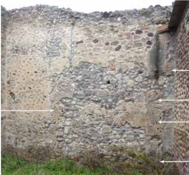
Fig. 10. Wall adjustment closing the boundary towards the House of the Greek Epigrams, viewed from courtyard V 1,23l in the North House of Caecilius Iucundus (south side of boundary). Note the frequent use of Sarno limestone ashlars and fragments within the adjustment. The arrows highlight some of the larger pieces. The full extent of this adjustment covers the space indicated between the arrows in Fig. 3. Photograph: Göran Kindström. Feature highlights: Henrik Boman.
