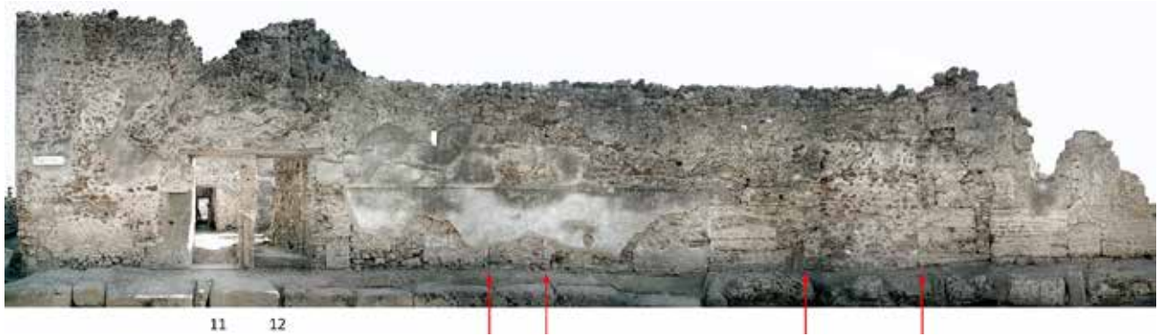
Fig. 15. North façade of the House of the Greek Epigrams (V 1,18.11.12). The arrows indicate two walled-up entrances attributed to the Northeast Building (the larger primarily diminished in width, then walled-up). See also Fig. 8. Photograph & orthomosaic: Hans Thorwid. Feature highlights: Henrik Boman.
