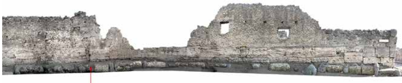
Fig. 17. North façade of V 1,13 along Vicolo delle Nozze d'Argento (a caupona in AD 79). The well-fitted, heavy ashlar of the lower part of the wall represent the oldest building technique ( opus quadratum ) evidenced in this insula. The arrow indicates the position of the pillar suggested as the return of the original north border of the Northwest Property. Photograph & orthomosaic: Hans Thorwid. Feature highlight: Henrik Boman.
