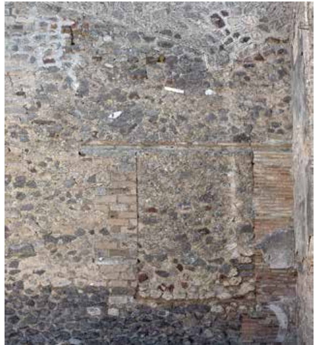
Fig. 12b. Walled-up window of east triclinium (later V 1,26o) opening towards and viewed from courtyard V 1,23l (see also Fig. 13). Photograph: Hans Thorwid.
