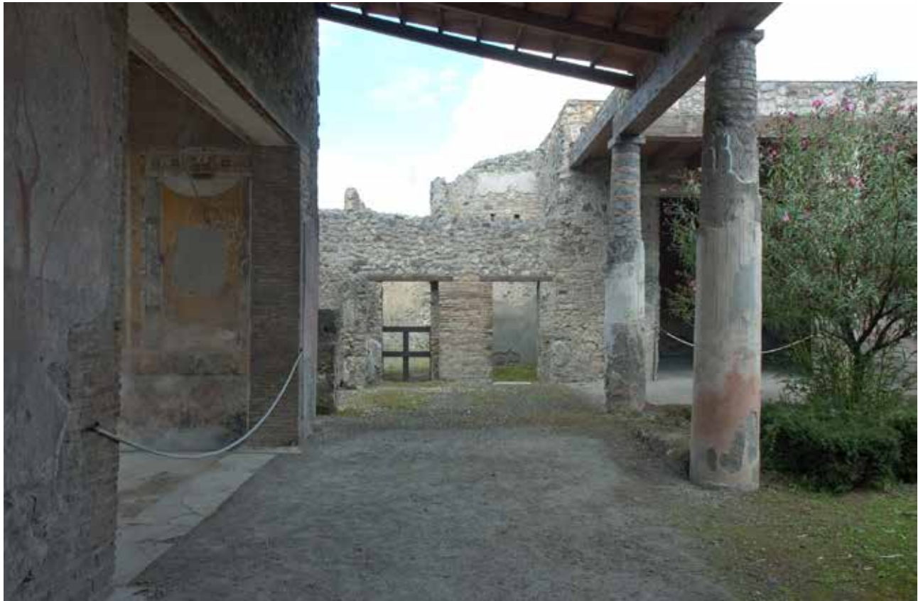
Fig. 33. Wall section in opus vittatum mixtum, support to masonry bridging two openings in the former boundary. View from the west garden portico of the South House of Caecilius Iucundus. The west doorway (left in image) opens on the corridor (V 1,23l') leading to open courtyard (V 1,23l) of the North House; the east doorway is the entrance to the new room (V 1,26n) built to flank the large triclinium V 1,26o (previously the east triclinium of the northern building). Photograph: Hans Thorwid.
