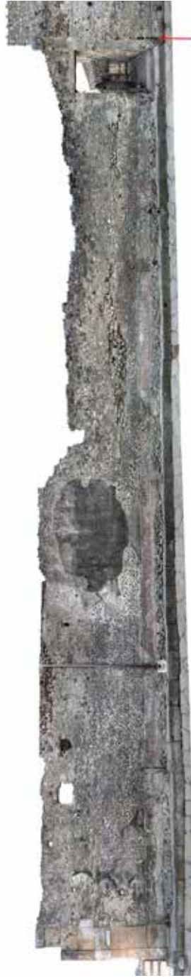
Fig. 2. East perimeter of Insula V 1, façade towards Vicolo di Cecilio Iocundo. Changes in stone material (indicated by arrows) mark the boundaries of four properties. Photograph & orthonosaic: Hans Thorwid. Feature highlights: Henrik Boman. The arrow between V 1,7.9 and V 1,26 is shown twice.
