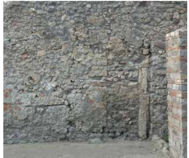
Fig. 11. North atrium wall of the North House of Caecilius Iucundus (V 1,23b). Note the Sarno limestone ashlars: to the right used as a door-jamb of a later walled-up doorway; to the left bridging a foundation fragility (latrine pit dug on the opposite side of the wall). Fragments are present as well. Photograph: Hans Thorwid.
