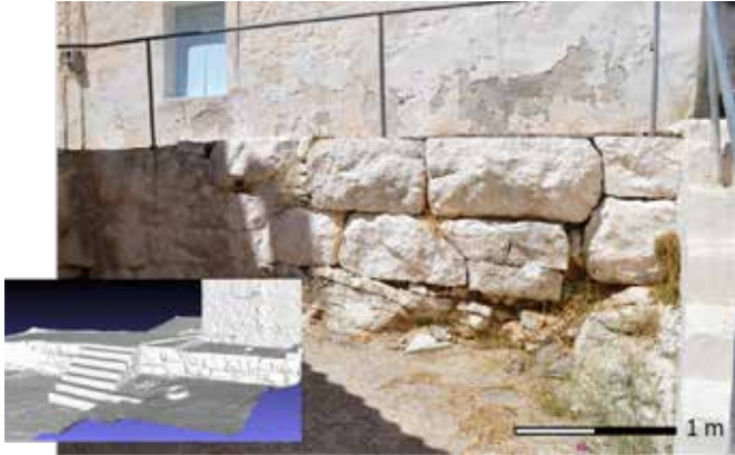
Fig. 15. Section of a stone socle for a mudbrick city wall on the south side of the Pron (western part, Fig. 3.17). View from the south. Photograph by Henrik Gerding, 3D rendering by Stefan Lindgren.
