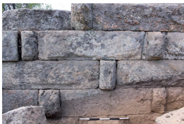
Fig. 6. Hekatomnid header-and-stretcher masonry of the central tower.
