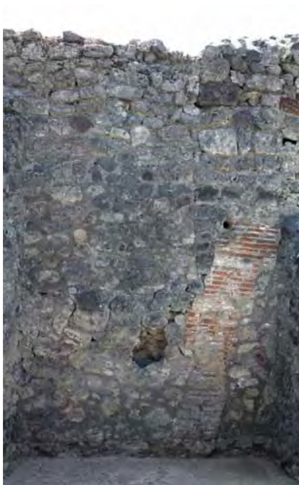
Fig. 23. Brick stitch repairing a fissure in the facing of the south wall belonging to the rear shop (b) of taberna V 1,24. By Hans Thörnid.
