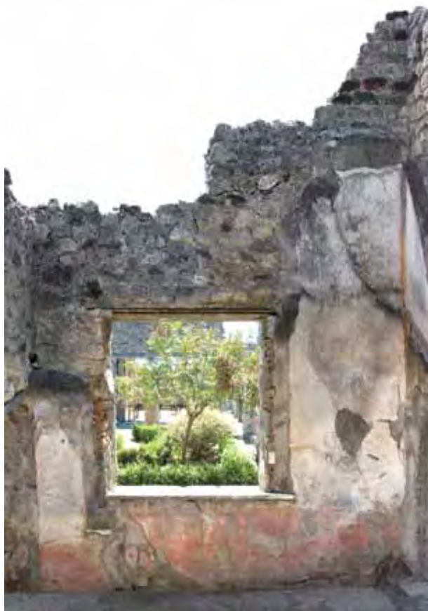
Fig. 26. Window with garden view. West wall of room s of the South House of Caecilius Iucundus . Note the sunken S part of the wall and the broken window-sill. By Hans Thornwid.
