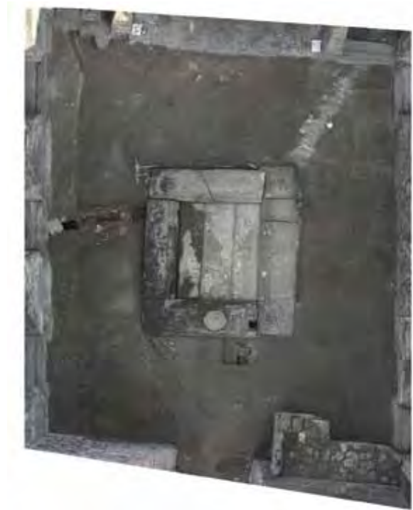
Fig. 28. Atrium floor of domus V 1,3. Note the water lines, the distribution box and the drains. North towards the top of the picture. By Hans Thorvid.
