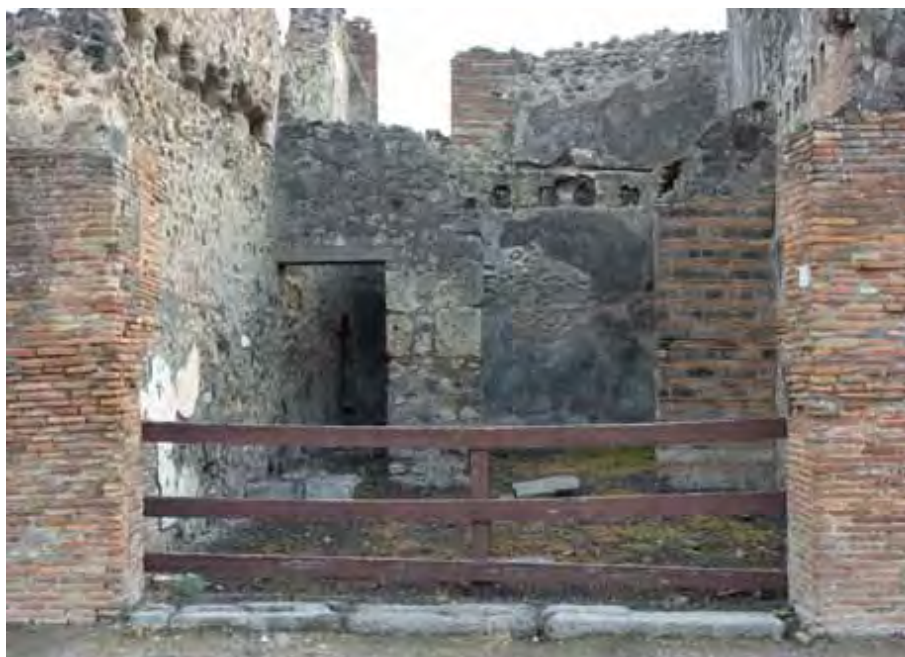
Fig. 30. Taberna V 1,31. Looking east. Note the two structures inside this space: the base of the staircase leading to the second storey situated against the north wall and the cistern mouth. The mouth itself is unfortunately mostly covered by the fence, but the cover stone demonstrates its central position in the floor of the front shop. By Hans Thörnwid.
