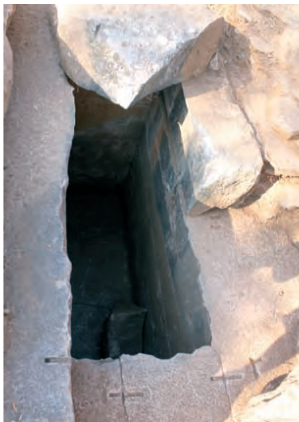
Fig. 86. Pi-shaped clamps on the top of the north wall of the main chamber.
