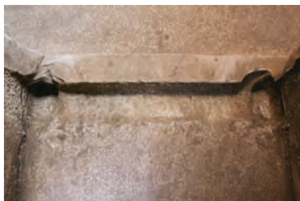
Fig. 79. The threshold block for the doorway between the vestibule and the main chamber, seen from the chamber.
