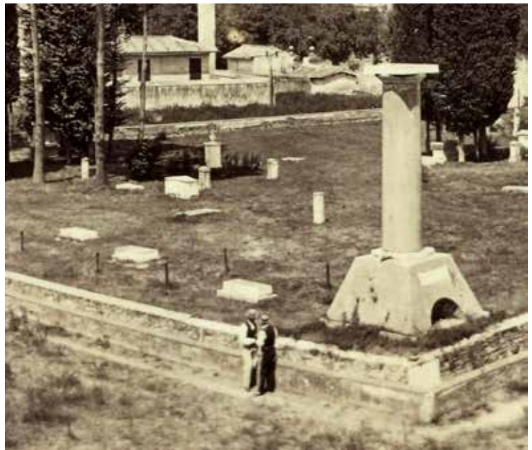
Fig. 3. Detail of Fig. 2 showing alignment of three ledgers and five wooden posts.
